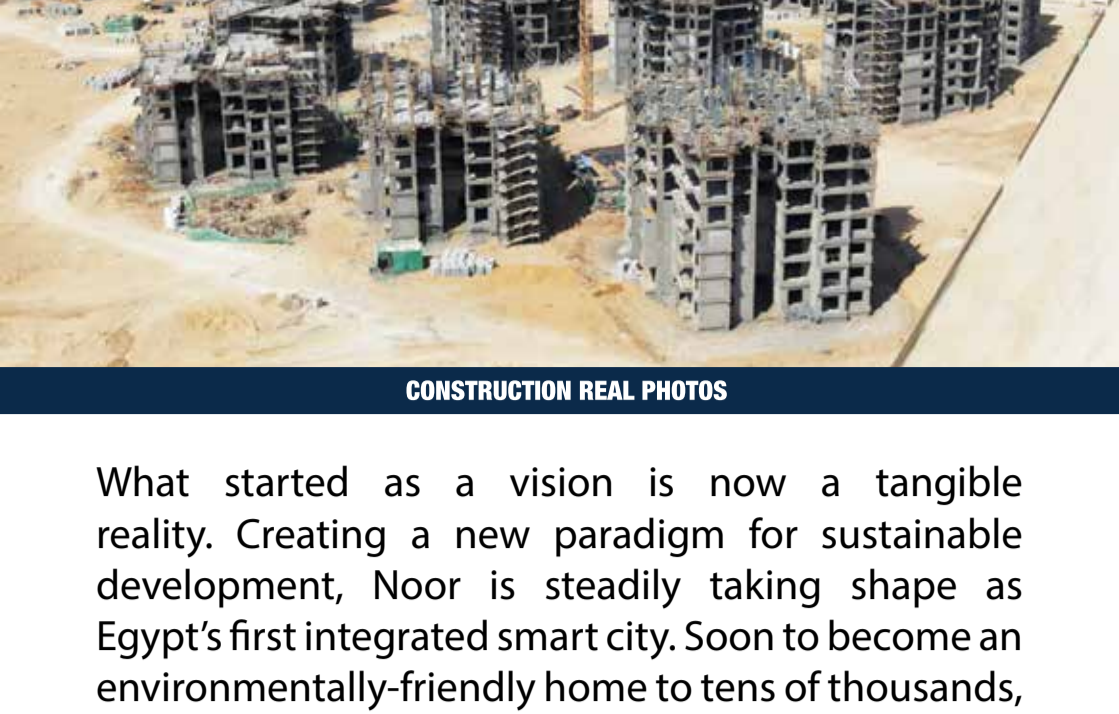
CONSTRUCTION REAL PHOTOS
